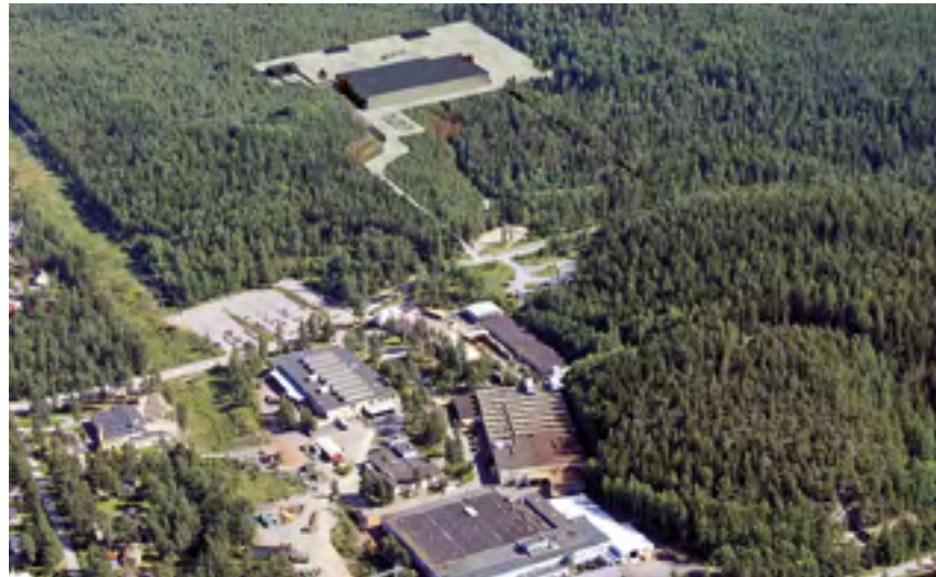
The new plant covers a total area of 9,200 square metres, including 6,600 square metres of heated area. The new plant can be seen at the top of the picture.
